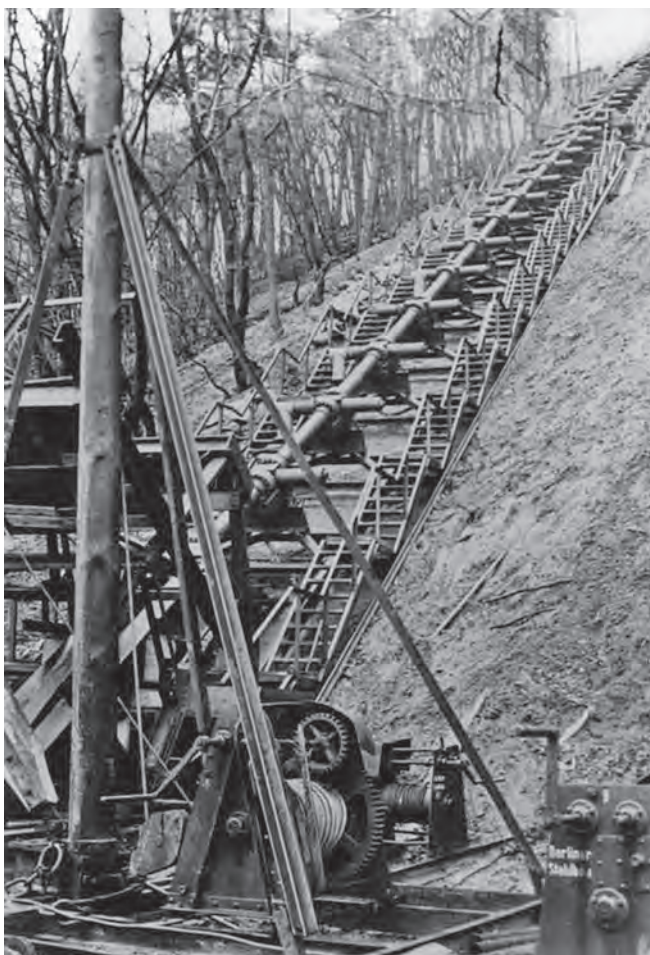
Prototype Gun Poland 1942 - An early supergun prototype at the Baltic test site, side charges arranged transversely; this was later revised into a more powerful slanted arrangement
